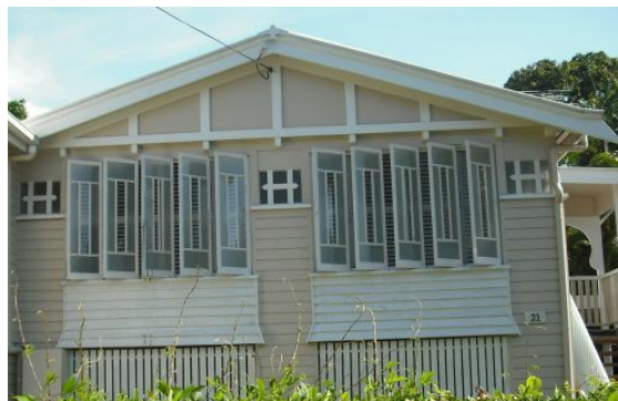
Figure SC6.2.3.15 Illustrates an example of five vertically proportioned casements located under the apex of a gable projection
