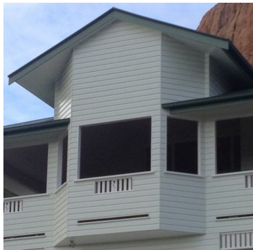
Figure SC6.2.3.21 Illustrates new works using manufactured cladding in imitation of traditional lightweight materials
